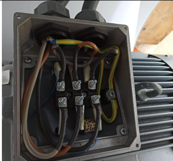
Photo 9. Motor Connection
