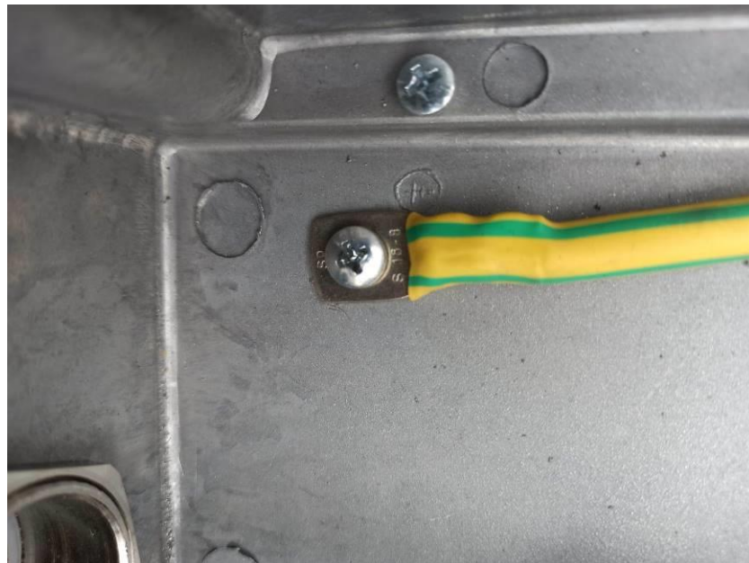
Photo 8. Earthing Connection
